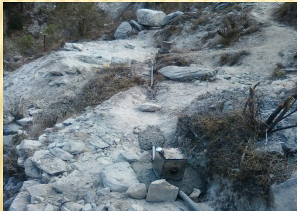
Piezometer wires to JCB within GI Pipe
