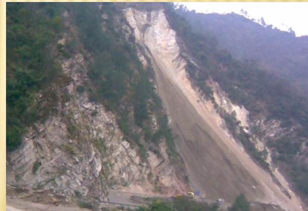
Kaliasaur landslide on Rishikesh – Badreenath Route
