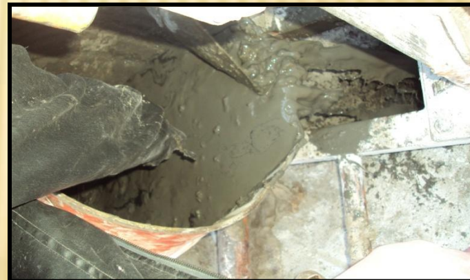
Filling of Borehole with cement Slurry
