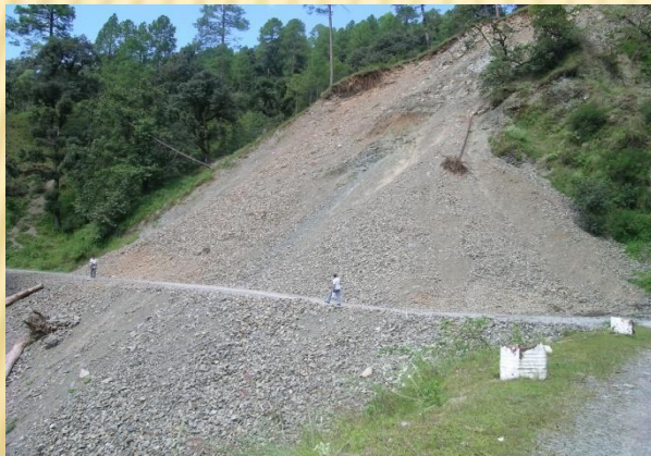
Dharasu – Yamunotri Route Landslide
