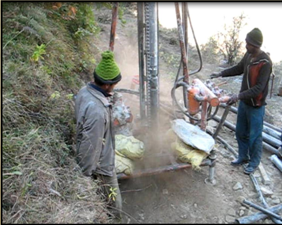
Process of Drilling
