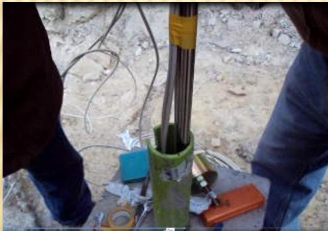
Wires held together with Gauge Tube
