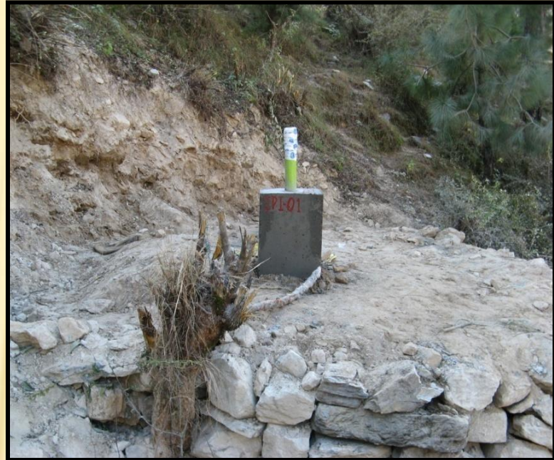
Platform created around Casing
