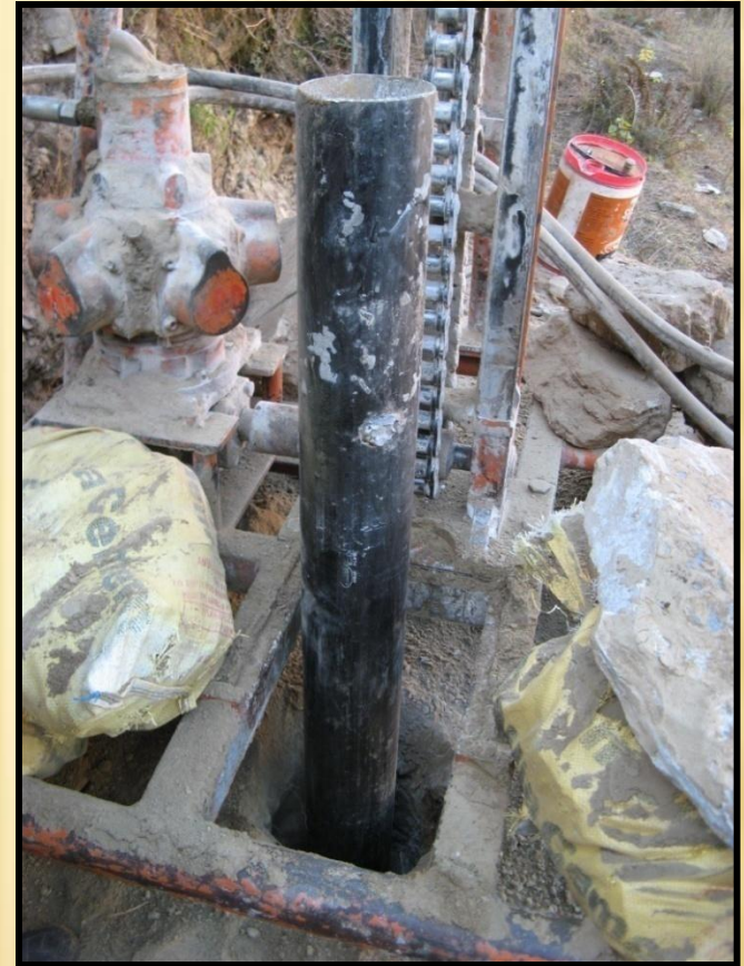
Installation of MS Casing
