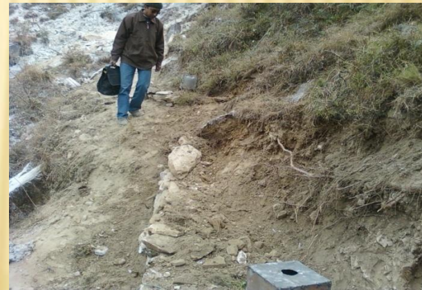
Pipes buried inside soil
