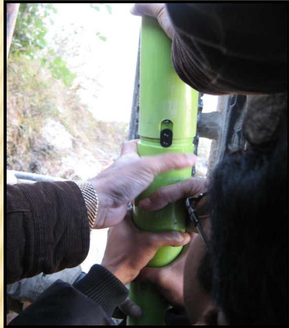
ABS Casing Connection
